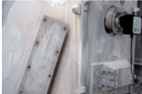
Electrofilter after a Calciner monitored by a Dynamic Opacity instrument
