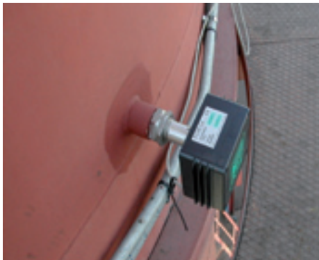
Crushing Plant Filter protected by an approved (TUV/MCERTS) advanced Electrodynamic® unit
