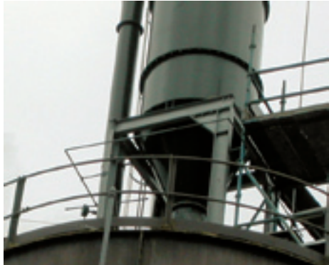
Silo Filter monitored by a networked Electrodynamic® sensor
