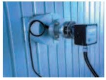
Dynamic Opacity monitor approved to TUV / MCERTS fitted to an electro-filter stack
