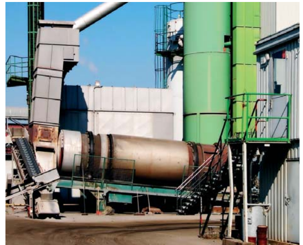
Application example: Rotary kiln within the chemical industry
